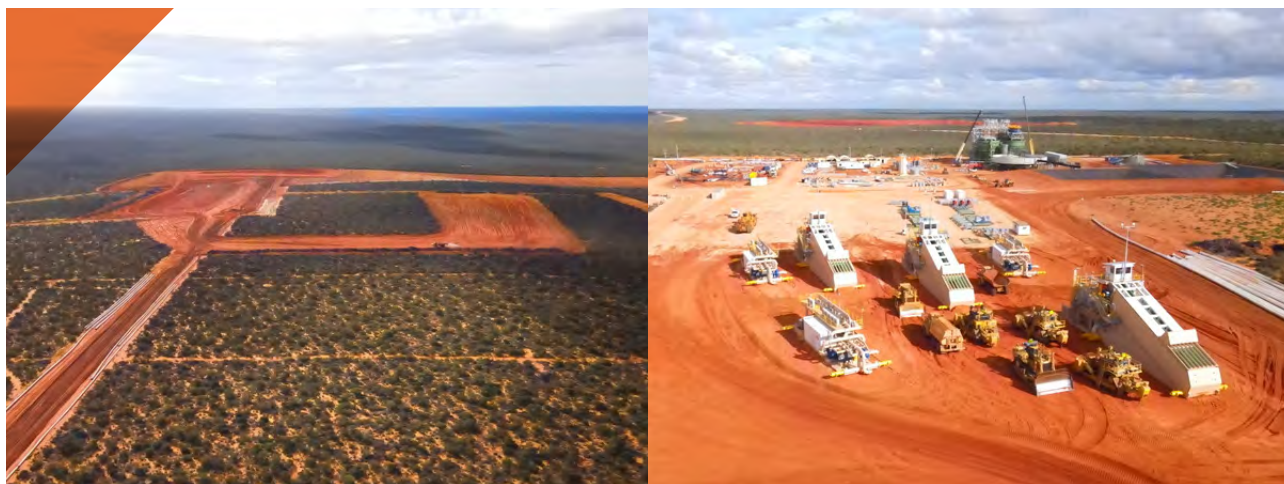
FIGURE 8: DEVELOPMENT OF OPEN MINE PITS & THREE DOZER MINING UNITS (DMU'S) READY TO BE MOVED INTO POSITION FOR MINING FIRST ORE
