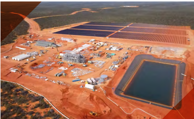
FIGURE 5: CONSTRUCTION OF COBURN'S HYBRID POWER STATION, MSP AND SUPPORTING INFRASTRUCTURE ADVANCING STRONGLY IN PARALLEL WITH WCP
