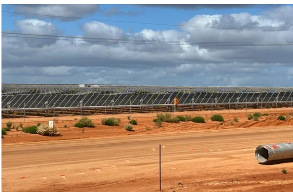
Figure 9: 11MW Solar farm + 4MW battery, designed to take full site power load under sunny conditions. BOO model via Pacific Energy.
