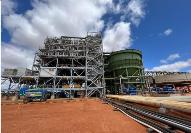
Figure 5: WCP spirals circuits – targeting 94% HMC grade
