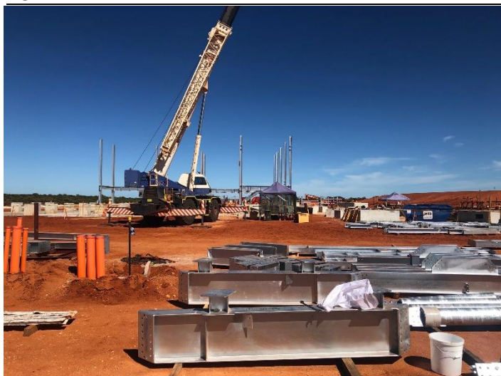
Figure 1: Wet Concentration Plant under construction
