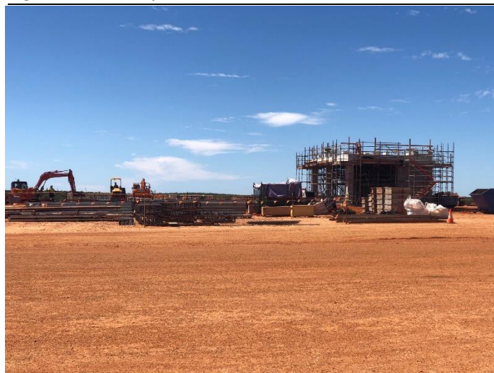
Figure 2: Mineral Separation Plant under construction
