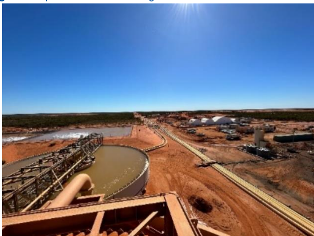
Figure 4: Pipework from the mining area into the Wet Concentrate Plant
